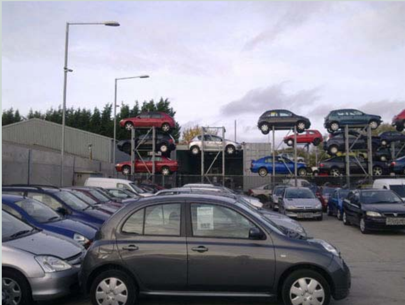
Fig 3 : View of the de-pollution building behind the existing car stacks facing north
