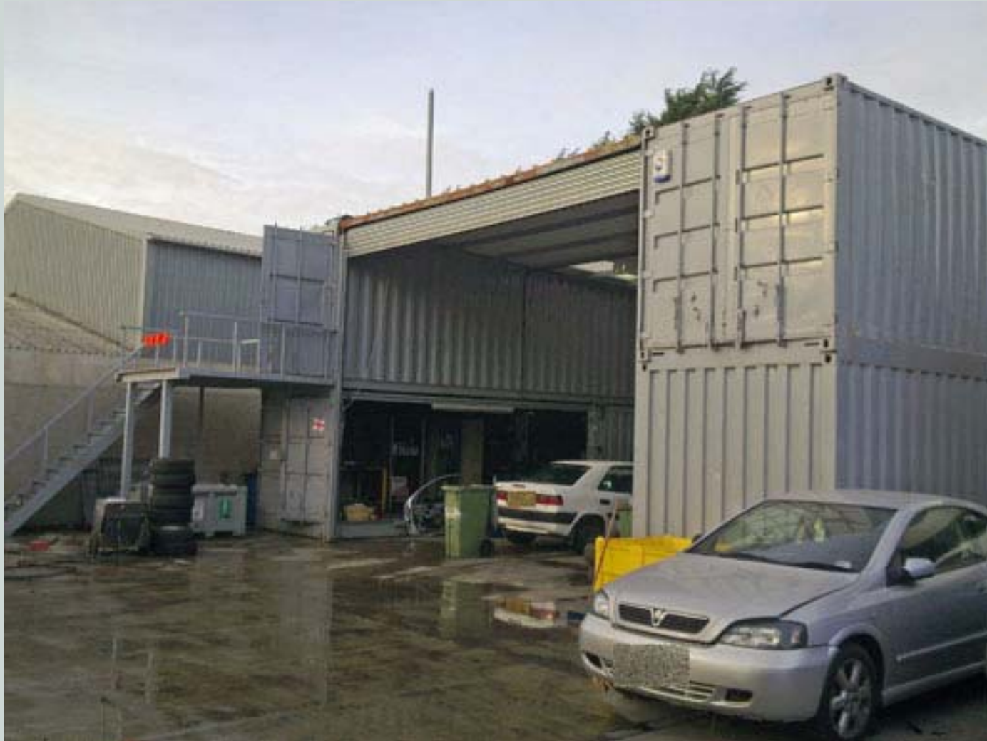
Fig 1 : View of the de-pollution building with Sanitrux storage building in the background facing west
