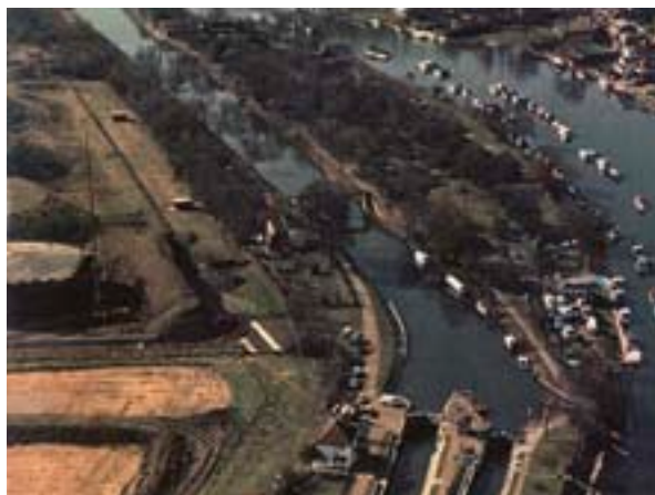
Aerial view of Sunbury Lock, looking upstream
