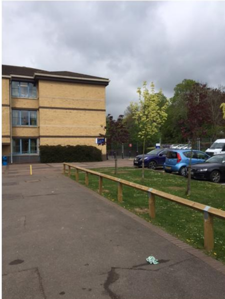
Figure 1 – Existing eastern elevation of main block to be extended
