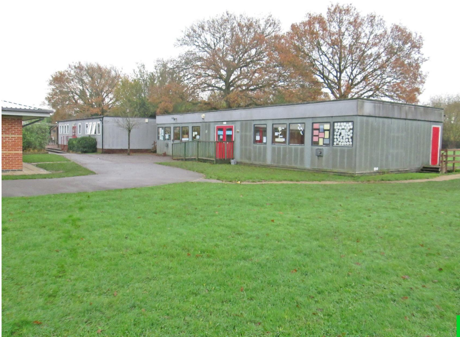
Figure 6 : Looking east towards the two modular buildings to be removed
