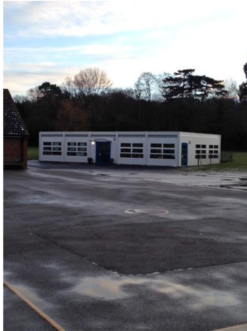
Figure 4 : Block 1 to be permanently retained as part of this application
