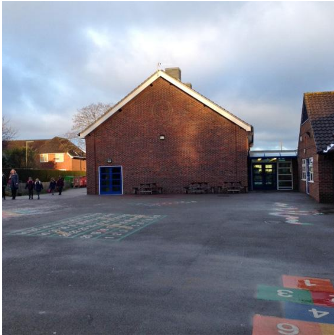
Figure 2 : Rear of existing hall to be extended
