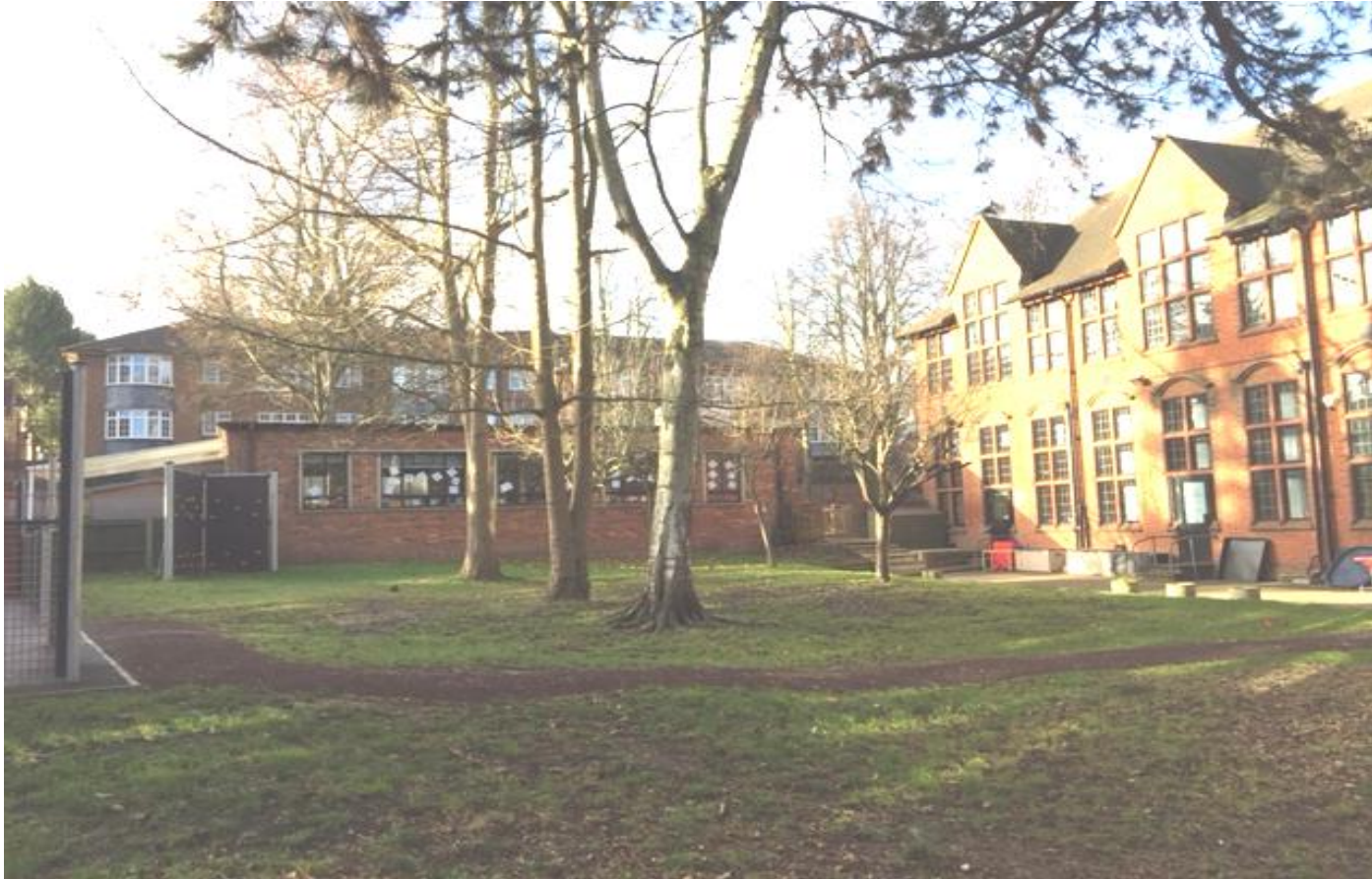
Figure 15 : Existing rear elevation showing nursery building adjacent (to be demolished)
