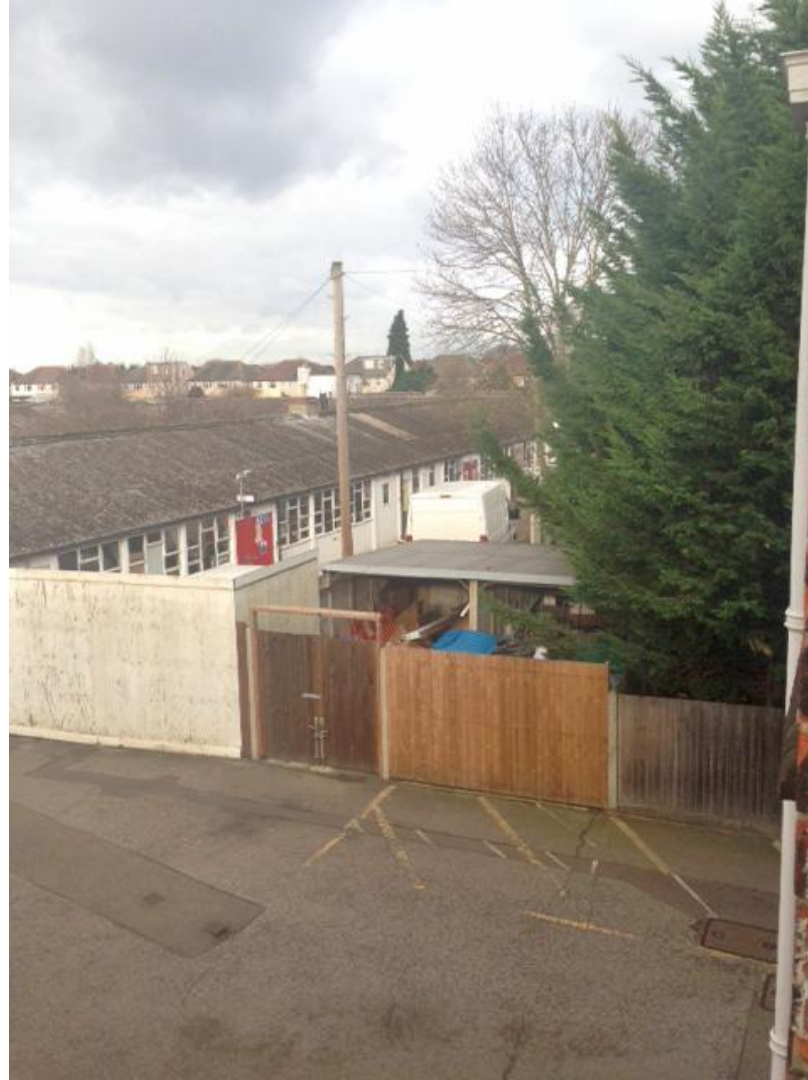
Figure 4 : Existing Gym maintenance building to be demolished
