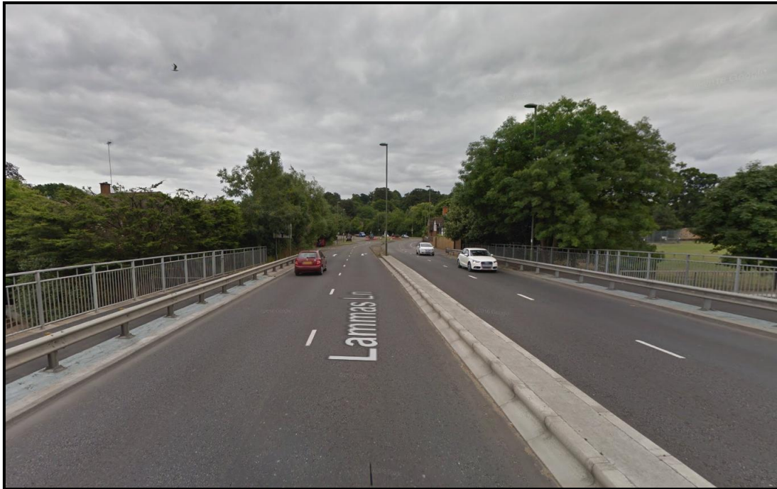
Figure 03: Lammas Lane westbound approach to roundabout with West End Lane.
