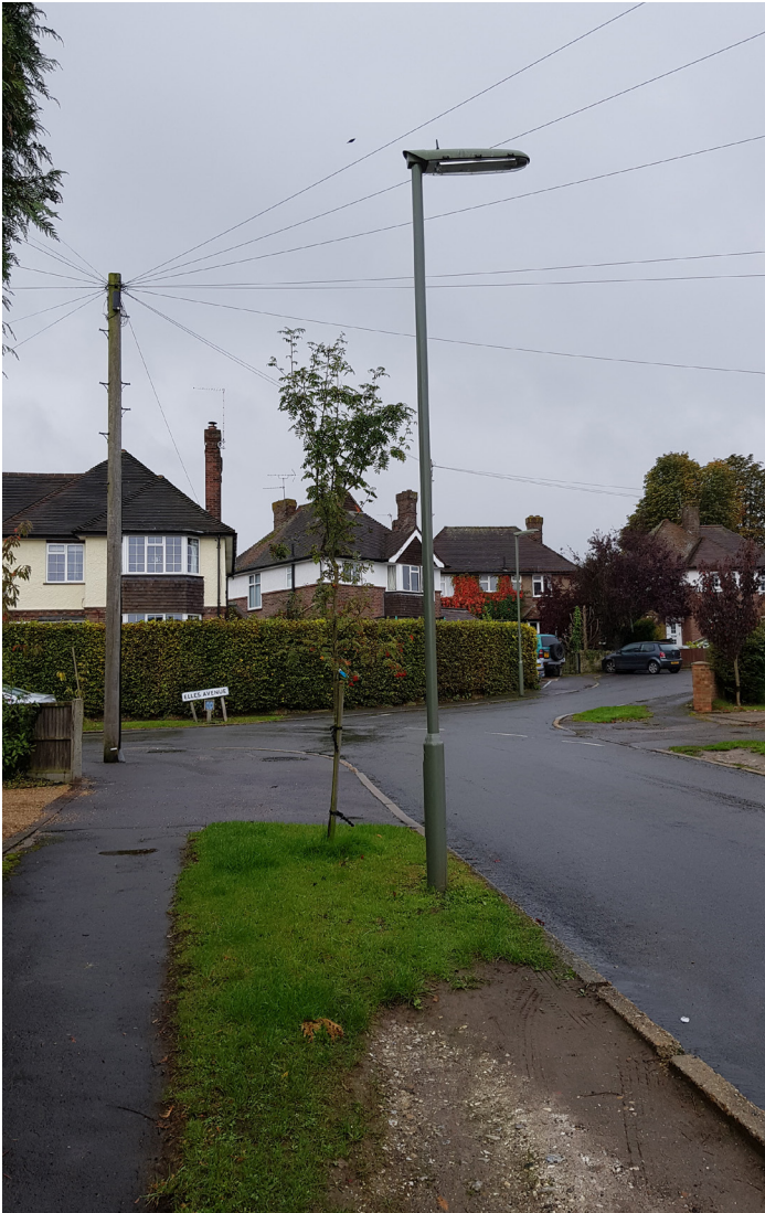
Rowan tree planted under telephone cables and too close to a street lighting column – this will cause issues in the near future.
