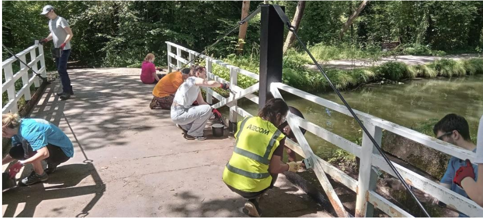
Volunteers painting Zebon Copse swing bridge
