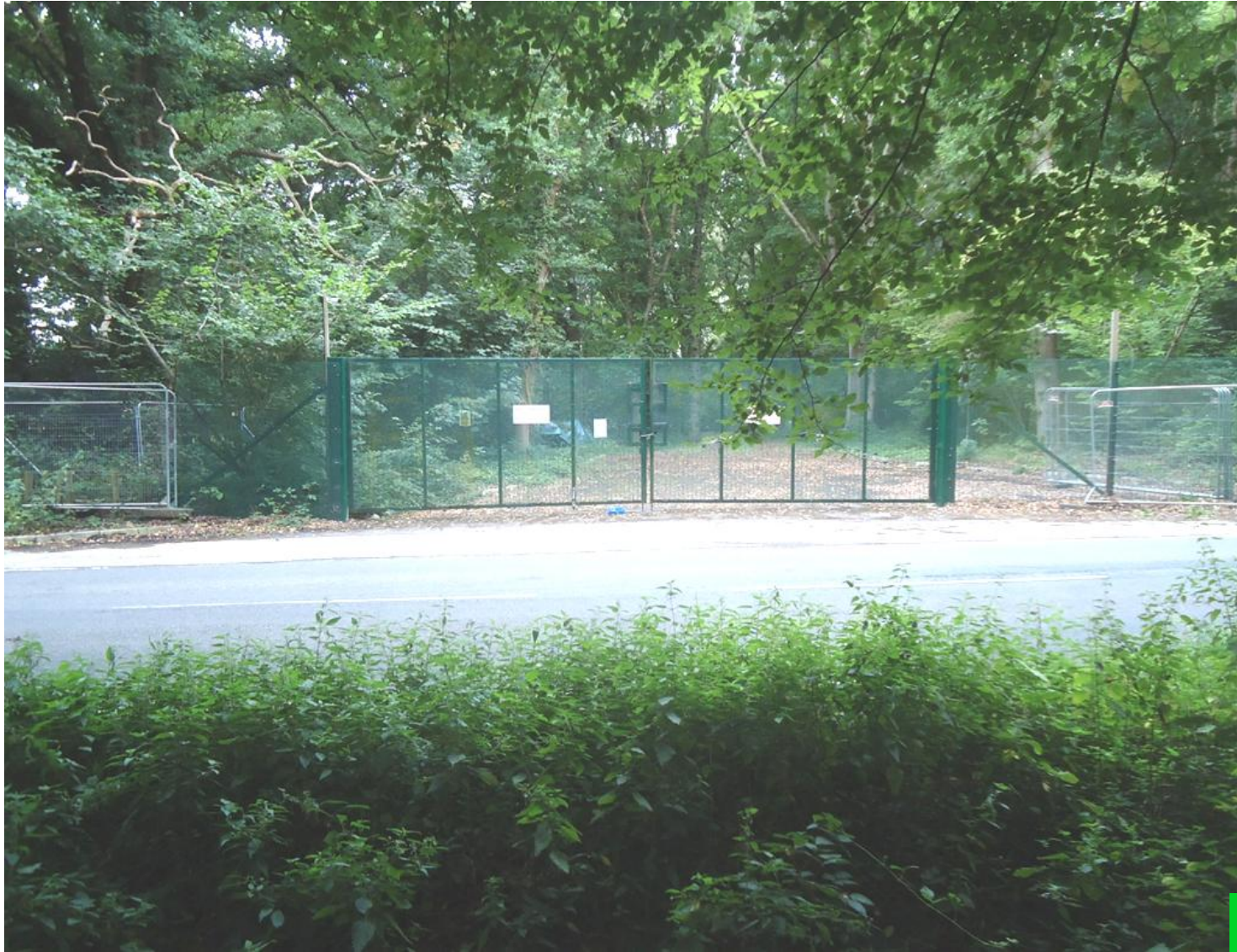
Photo 3 : The existing wellsite access on Horse Hill
