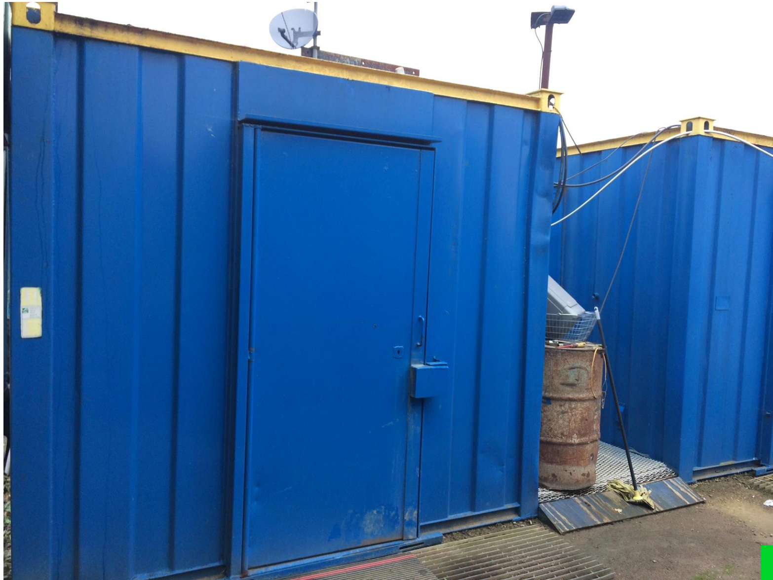
Figure 1 :- Container Unit 1: Clothes Drying Room
