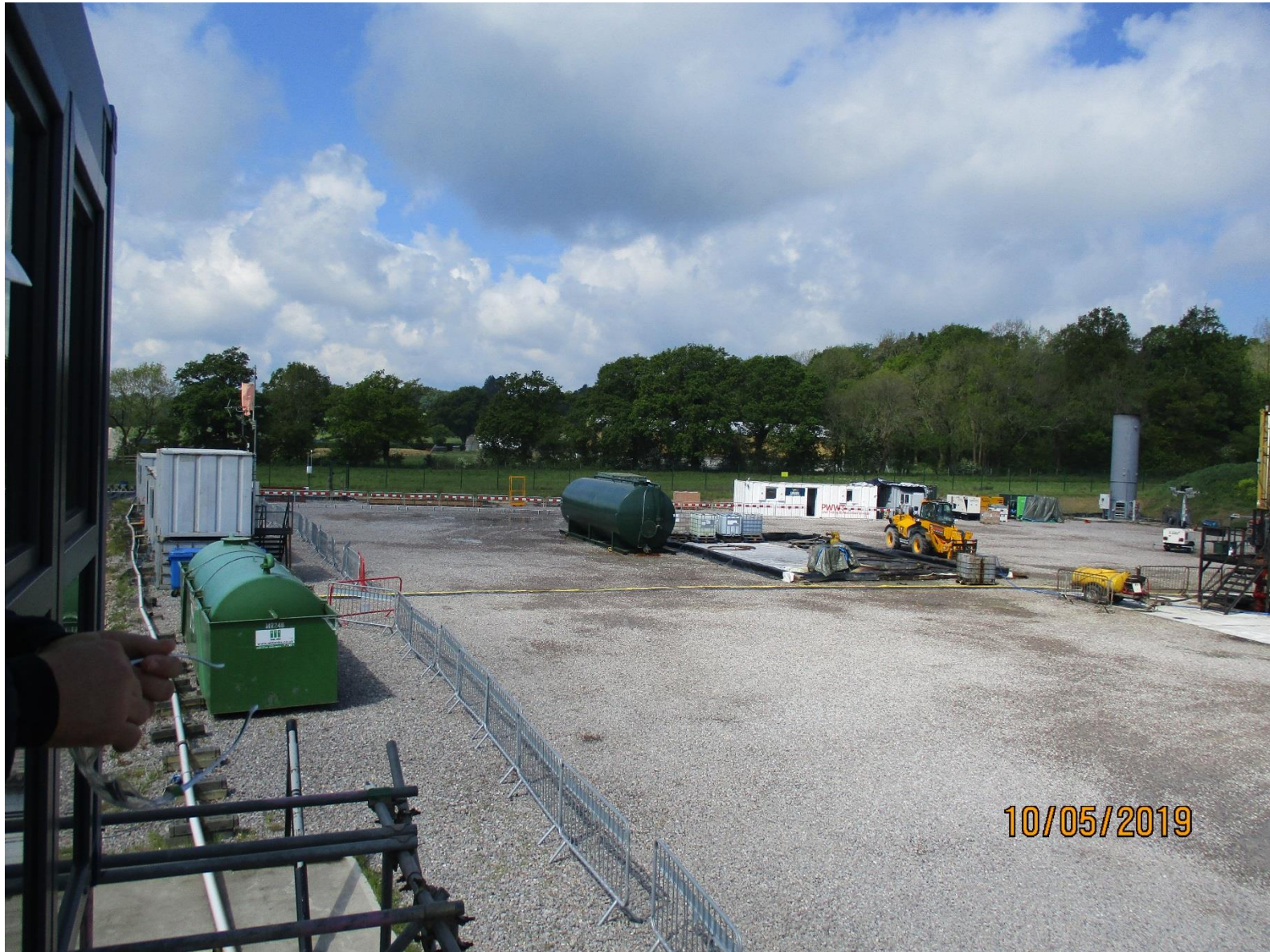
Figure 6 – The existing well pad western boundary
