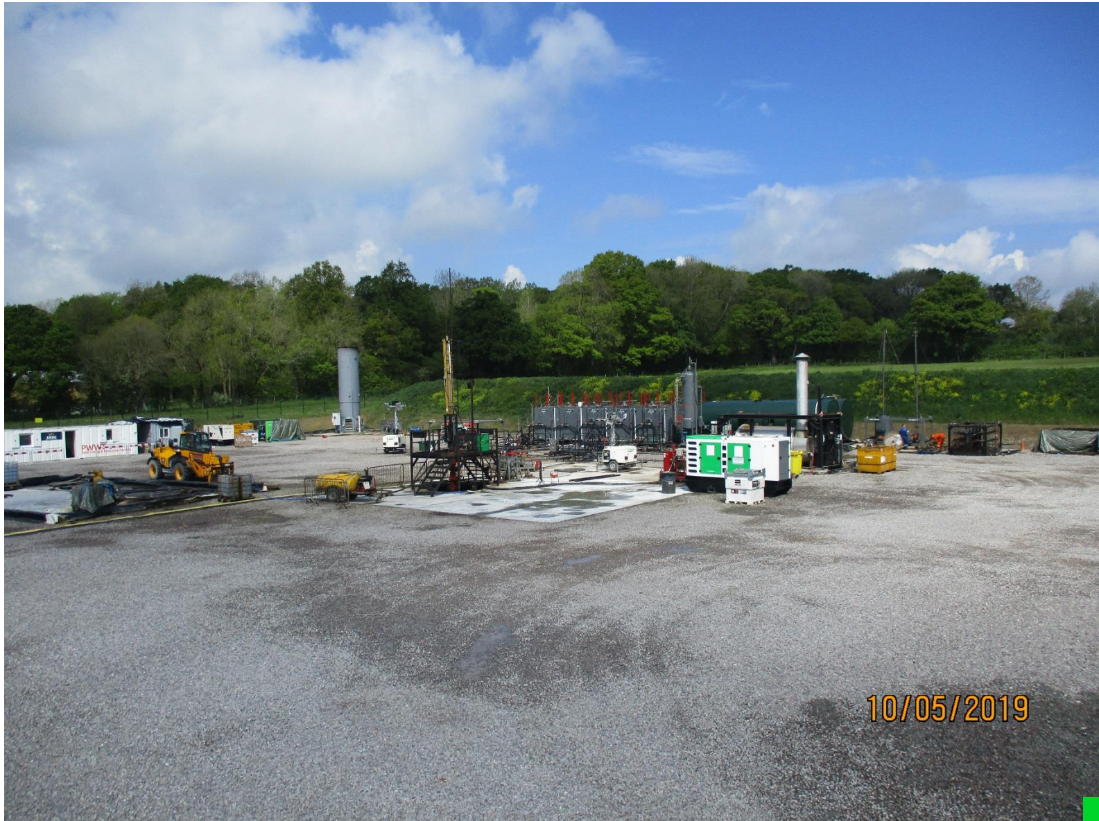
Figure 3 – The existing well pad viewing north west
