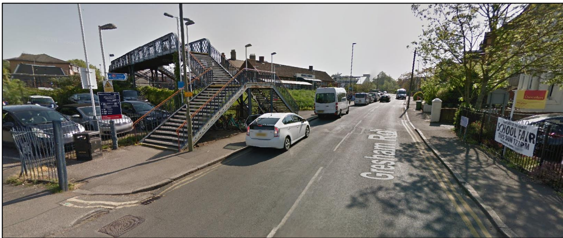
Figure 02: Middle of Gresham Road, by Staines Train Station.
