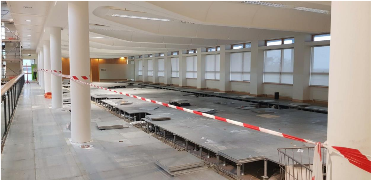
Infrastructure being completed
