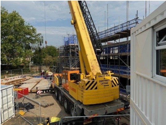
Image of the crane in position lifting the prefabricated roof panels from the ground to the roof at Fordway Centre in Ashford.
