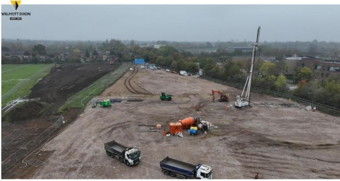
Image of construction vehicles working on stripping the site's topsoil and ground-cutting on Hopescourt School's permanent site in Walton-upon-Thames
