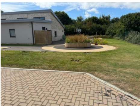
Image of the new 6th Form block at Woodfield School with external landscaping completed in Merstham
